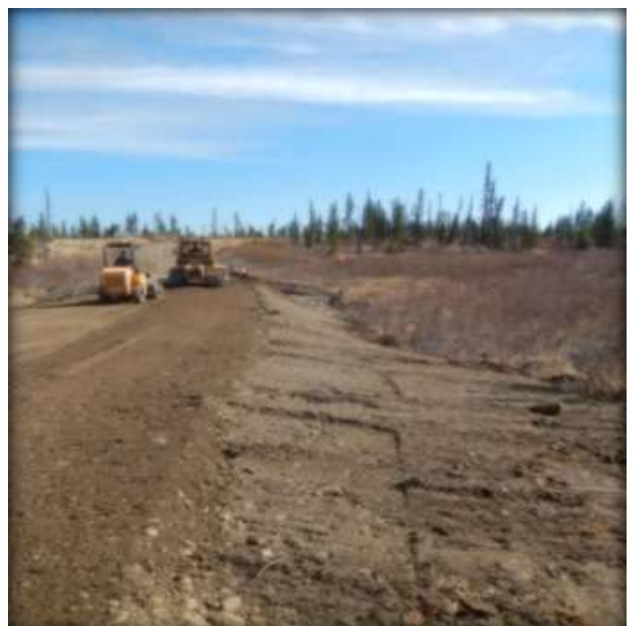
CSP Added Many Upgrades to NNAI Roadways
